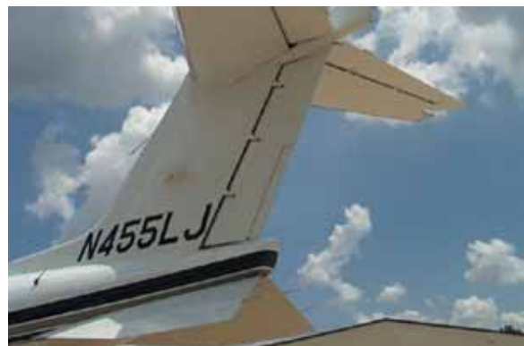
Figure 15a—V Stabilizer, Rudder, H Stabilizer, Elevator, Delta Fins, and Logo Lights (if installed) Condition, drain holes clear
