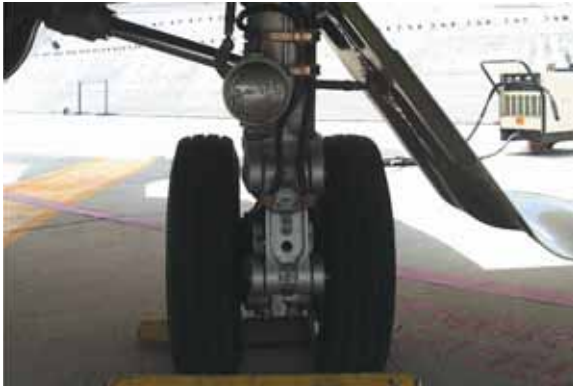
Figure 22b—Left Main Gear Check: wheel well—hydraulic/fuel leakage and condition; taxi light and doors—condition; wheels, brakes, and tires—condition; main gear strut—check proper extension
