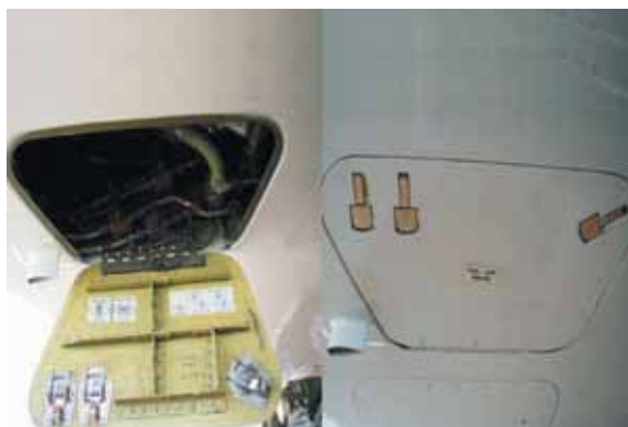
Figure 22a—Fuel drains and Access Door Drain if contamination is suspected and secure
