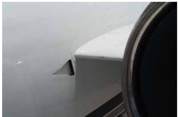
Figure 22e—Upper Fuselage, Fuel Vent Inlet Clear of obstructions and condition
